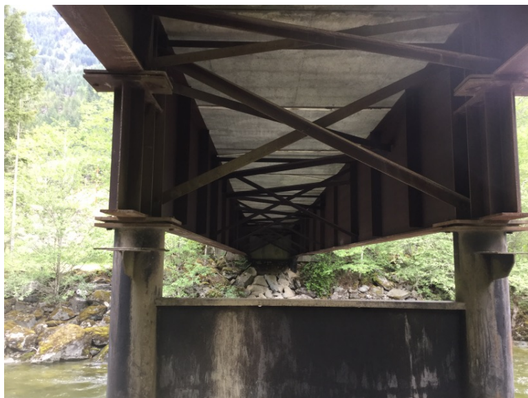
Main span superstructure
