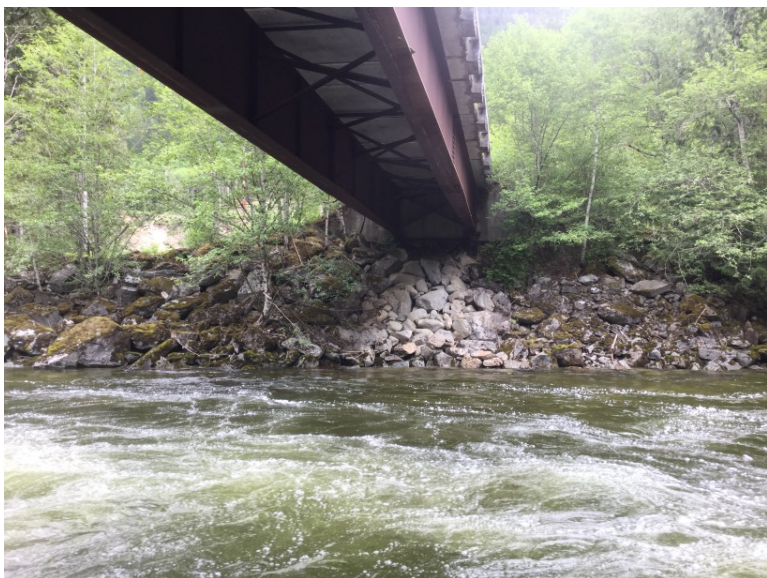
Left Bank Abutment when facing downstream
