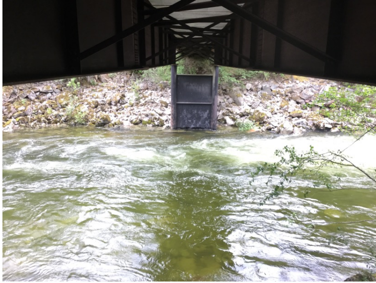
Right Bank Abutment when facing downstream
