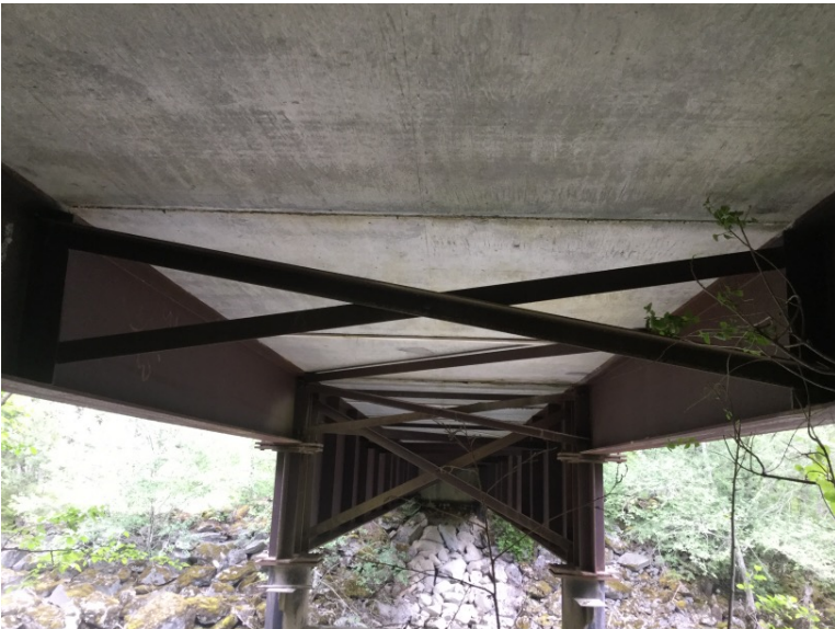
Jump span superstructure
