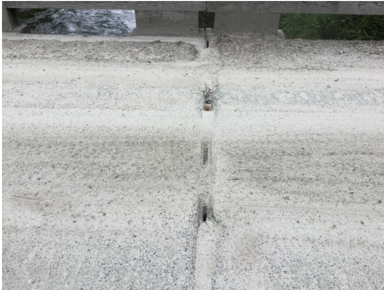
Span deck joint
